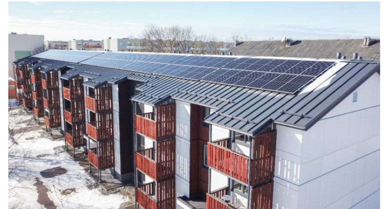
Nuotrauka: Kalle Kuusk, Tallinn University of Technology, Estonia Business and Innovation Agency presentation „Circular modular solutions in mainstream retrofit“.
